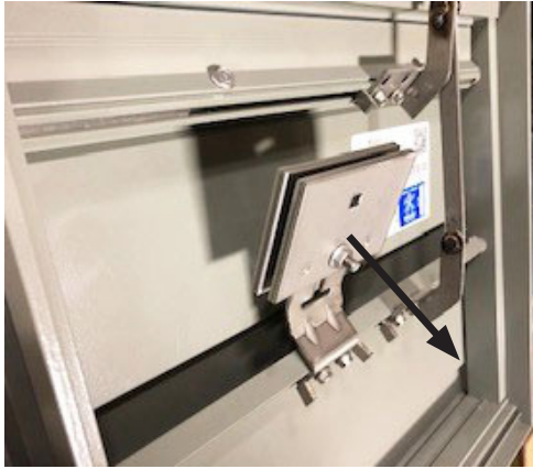
Bend counterweight mounting bracket away from blades.
